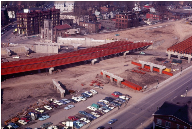
Insertion of Steel Placements, April 1967 (DOT)
